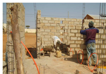
Building site - March 2008
